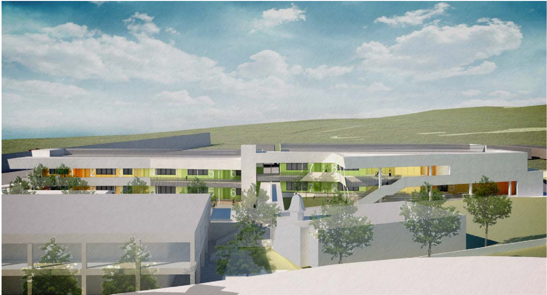
OVERALL PROJECT AERIAL VIEW
