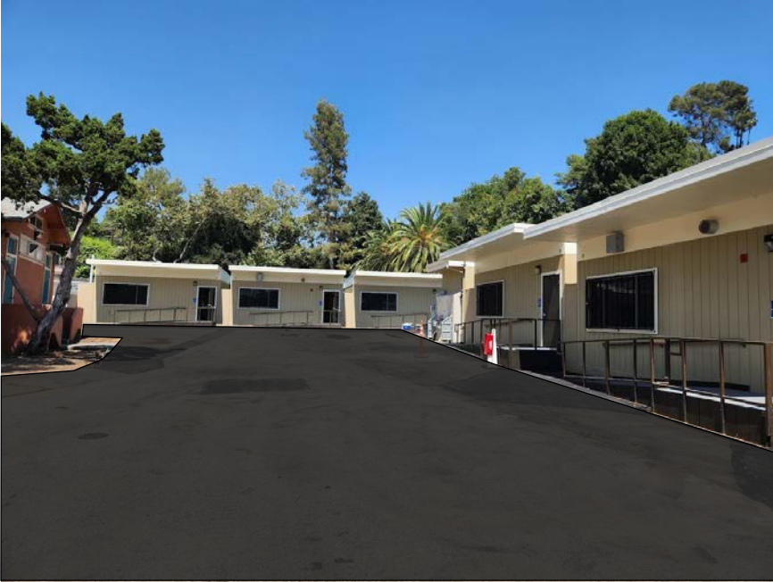
7 Interim Housing Units, Classrooms & Restroom 7 Unidades Temporales: Aulas y Servicios Sanitarios
